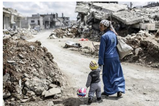
Damaged infrastructure in Syria due to civil war
