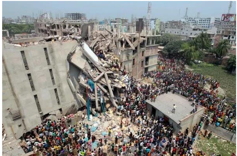
Scores Dead in Bangladesh Building Collapse
