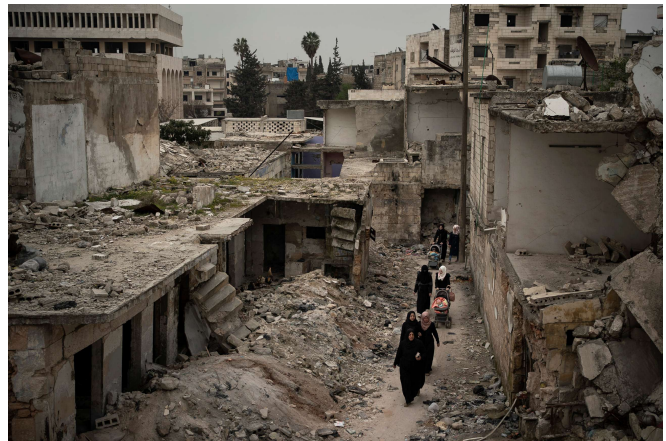
Civilians walking through a neighborhood heavily damaged by airstrikes
