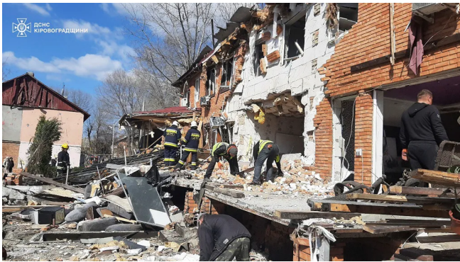
Image 3: Residential building damaged by armed drone attack in Ukraine
